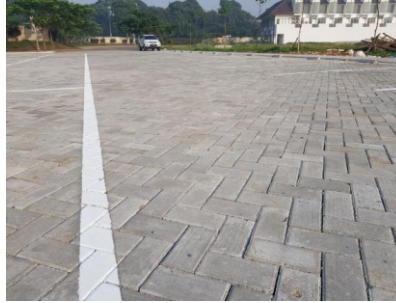
PT Wijaya Kusuma Construction (Binus Vida - Parking & Pedestrian)
